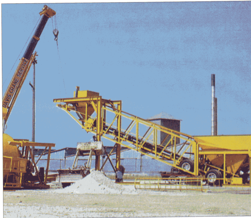
Main HSM truss module being lifted into place.
